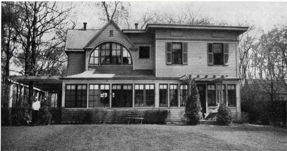
This well-built old house had a good location in a desirable neighborhood. Its ugly architecture, with the unrelated details and roofs and forms, suggested remodeling and modernizing as the only way out. The finished job is shown below.
