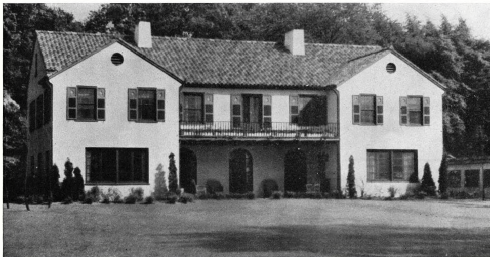
The left wing is all new. The enclosed porch with its row of windows was removed. Roofs were reconstructed. The second-story arched window was eliminated. The result is harmony and balance, and economically sound home ownership.
